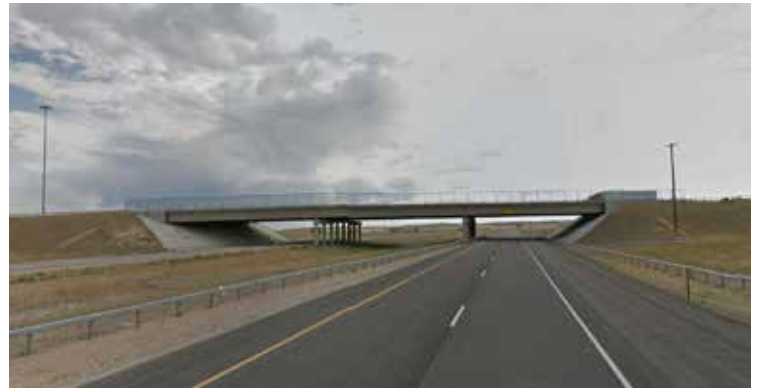
Figure 63: I-25 North looking northwest at Hat Six Road overpass in 2014
