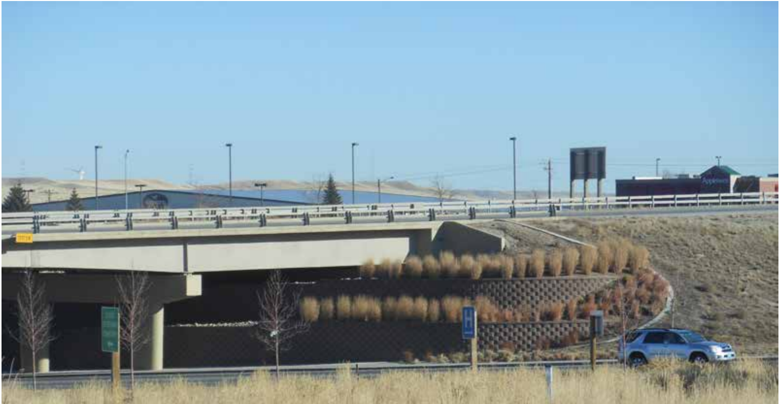
Figure 58: Wyoming Boulevard/Curtis Street Interchange enhancements in 2014
