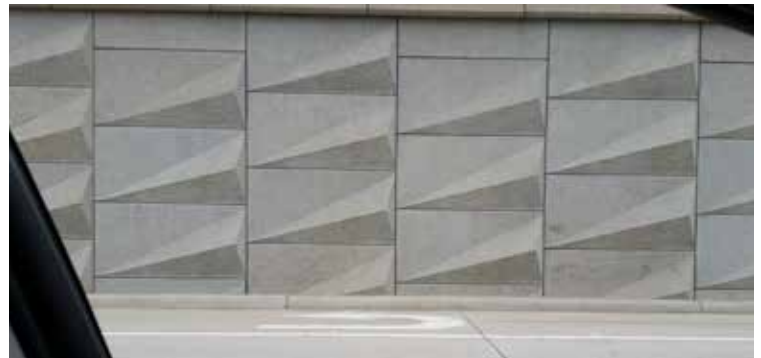
Figure 20: Example of a vertical abutment as a part of a MSE wall that features a 3D form liner within a narrow corridor
