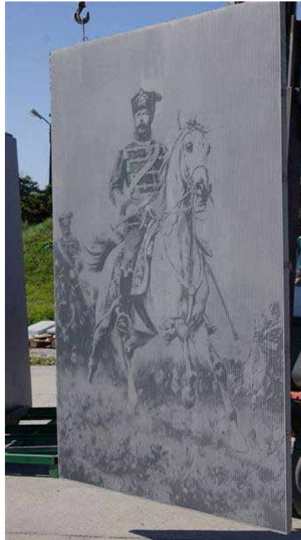
Figure 27: Photo-realistic concrete form liner technology
