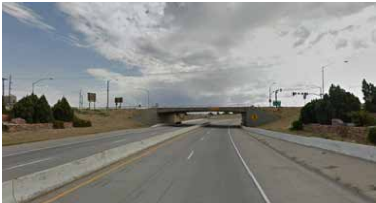
Figure 55: Bryan Stock Trail Overpass in 2014
