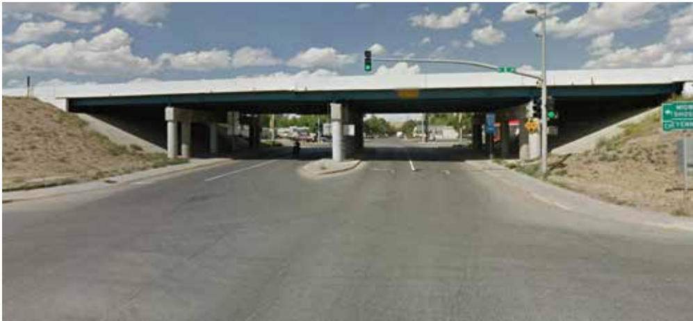
Figure 49: McKinley Street Underpass looking north in 2014
