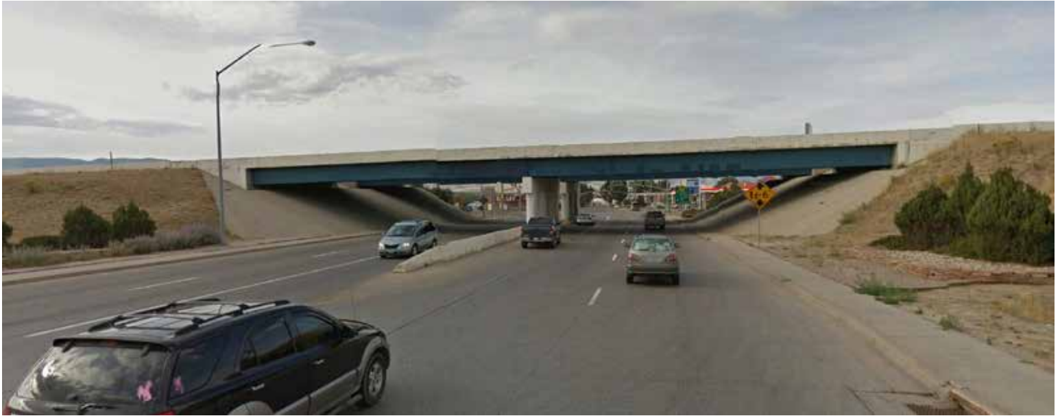
Figure 45: Poplar Street Underpass in 2014
