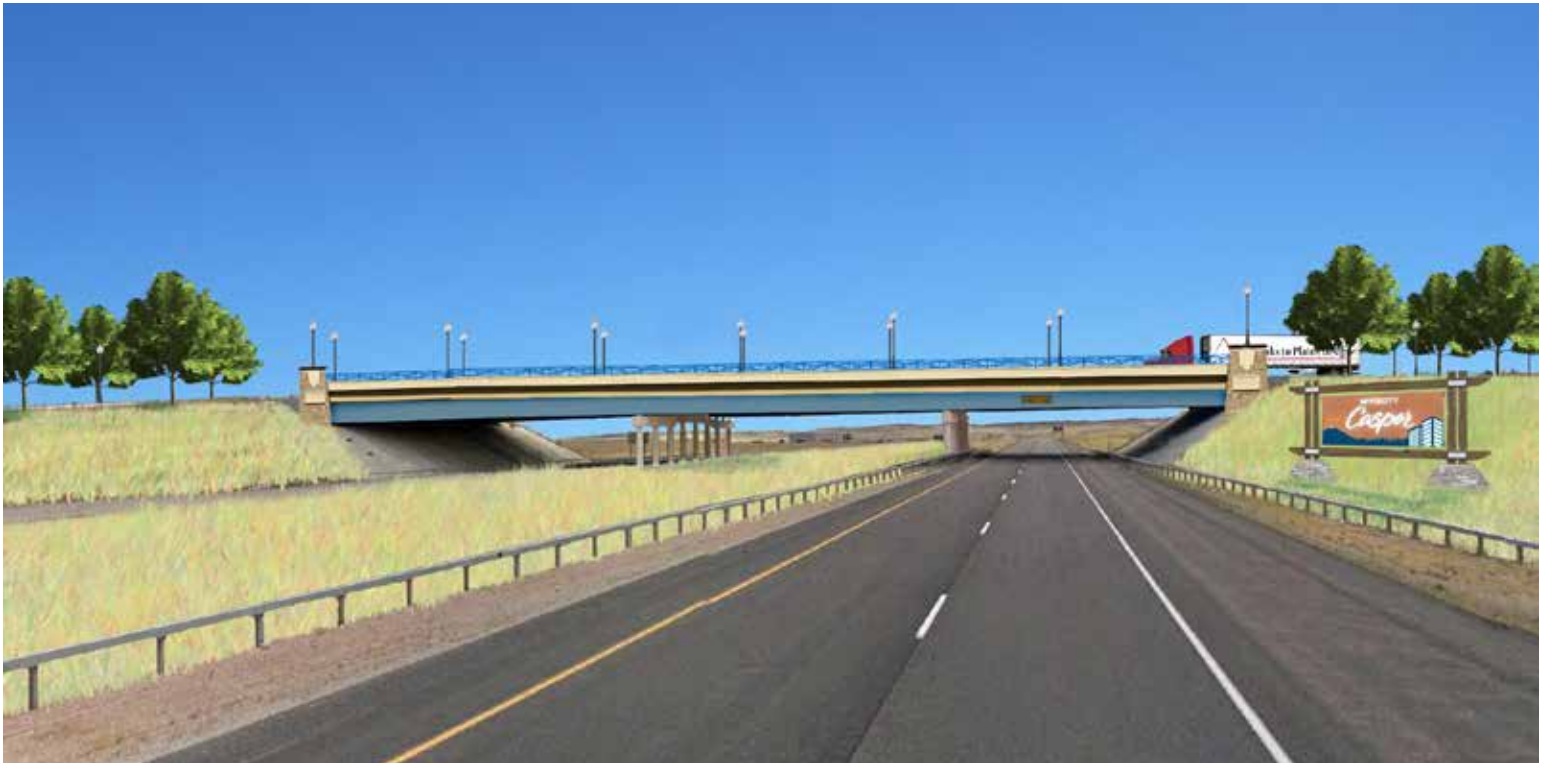
Figure 64: I-25 North looking northwest at Hat Six Road overpass
