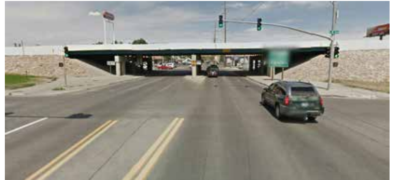
Figure 47: Center Street Underpass looking North in 2014
