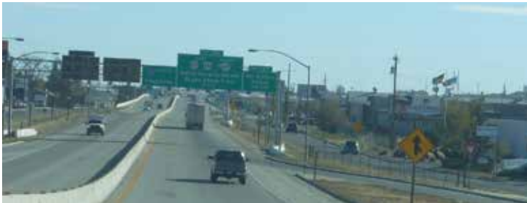
Figure 29: Regulatory and warning signs clutter up about 10 percent of this view approaching the McKinley Street exit
