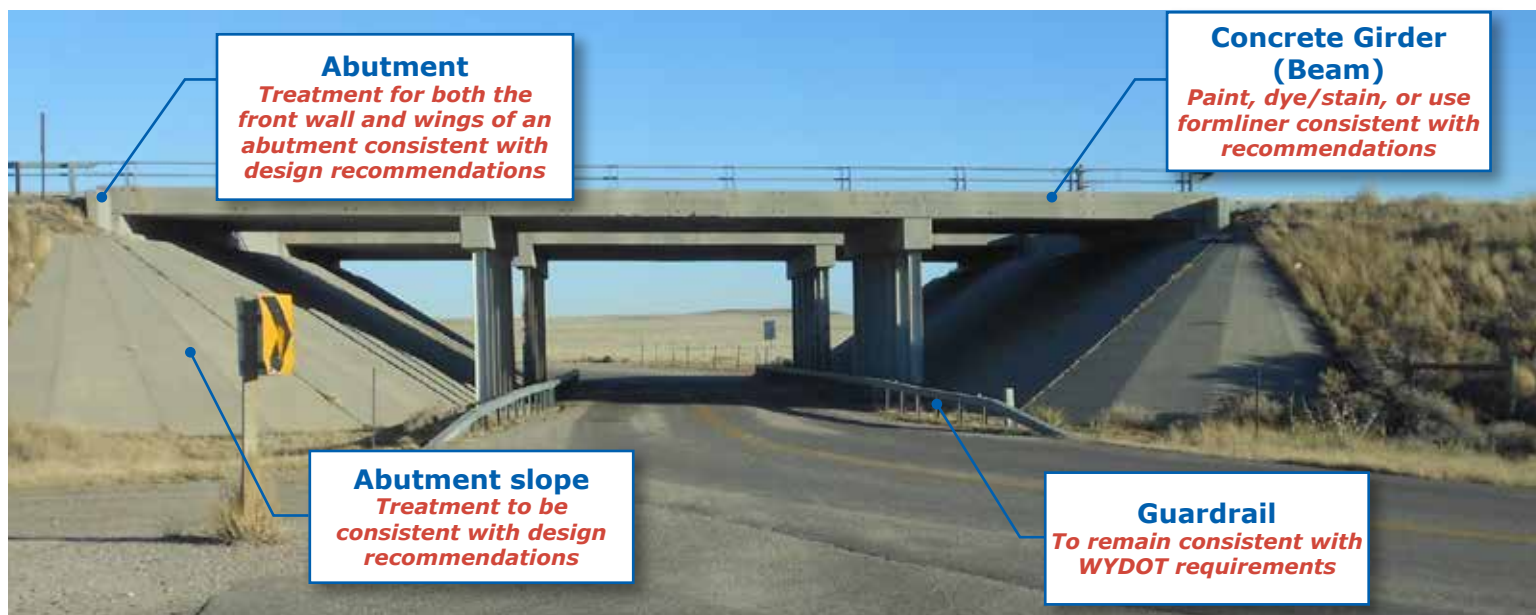
Figure 15. Typical elements of an overpass bridge
