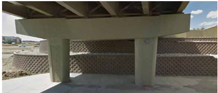
Figure 25: Wyoming Boulevard/Curtis Street pier with a concrete form liner application and terraced abutments
