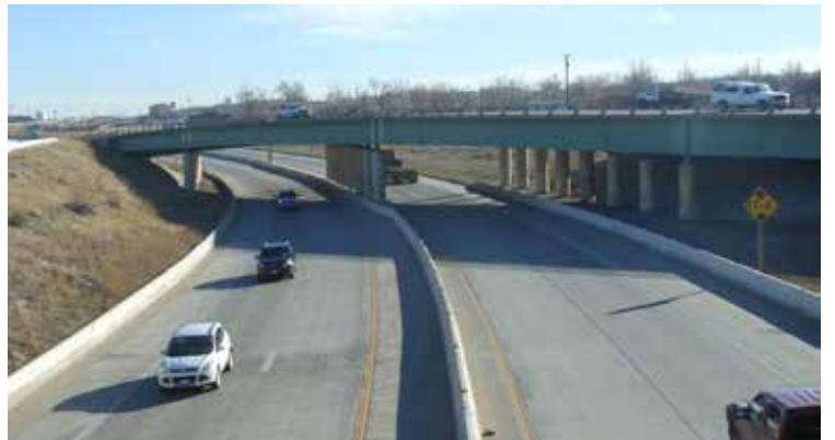
Figure 56: View to the east looking at Highway 26 (East Yellowstone) in 2014
