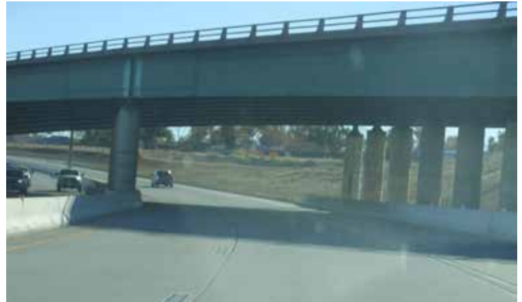
Figure 17: Example of a concrete girder system bridge
